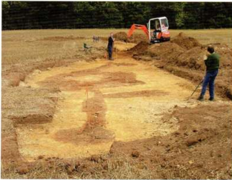
Left. Topsoil is machined off in an area next to the River Wharfe just outside Boston Spa, Yorkshire, where fieldwalking and geophysics have located an enigmatic site. A bizarre arrangement of pits and gullies was immediately revealed.
